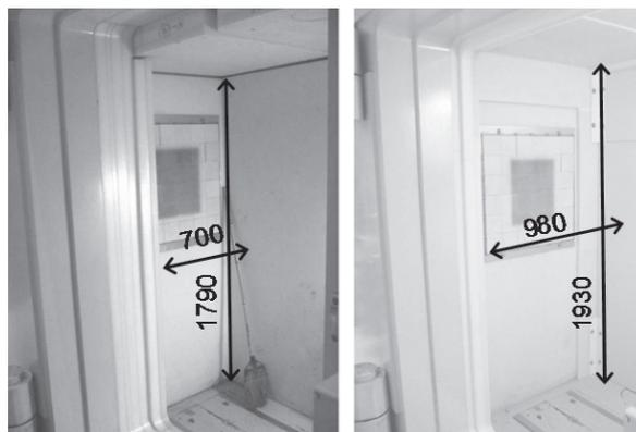
Figure 1: Inside view of TNRF-2 from the shielding door opening. Left side photograph was taken before the expansion work and right one after the work.
